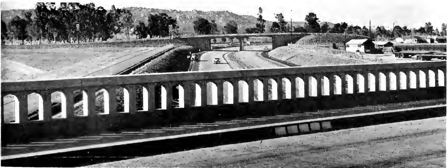
View of US 395 from Perris Boulevard Overcrossing looking north to D Street on-ramp
